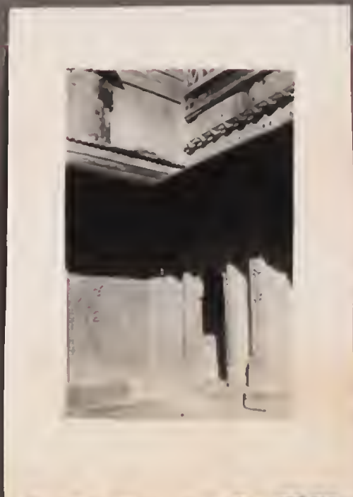
Interior of Palace in Zamboanga
